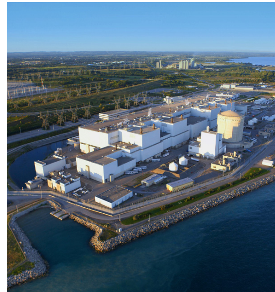
▲ In Ontario, refurbishment work at the Darlington Nuclear, Pickering Nuclear, and Bruce Nuclear all continue to employ hundreds of Teamster members with more work being proposed in the near future. Some of our members have worked for well over 20 continuous years at these facilities. Image credit: OPG
